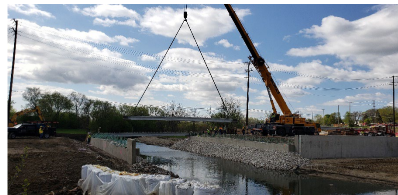
DOTD crews working to rebuild a bridge in suburban Cook County
